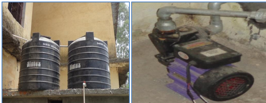
Installation of overhead tank (left) and Electric Motor fully made operational
